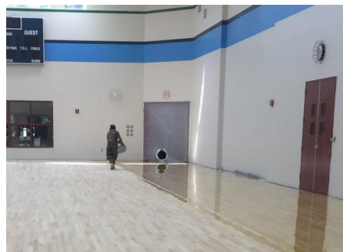
Finishing and Sealing New Gym Flooring
