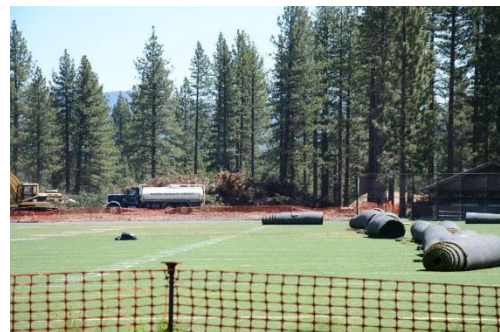
Early Construction of New Soccer Field
