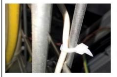
Scratch that! A repeat ask from TSO Not up to scratch From our colleagues in TSO, a request to check that if you're using cable ties, around making sure that cable ties are that you use the right tools to cut them off and make sure they've been left as safe as possible.
